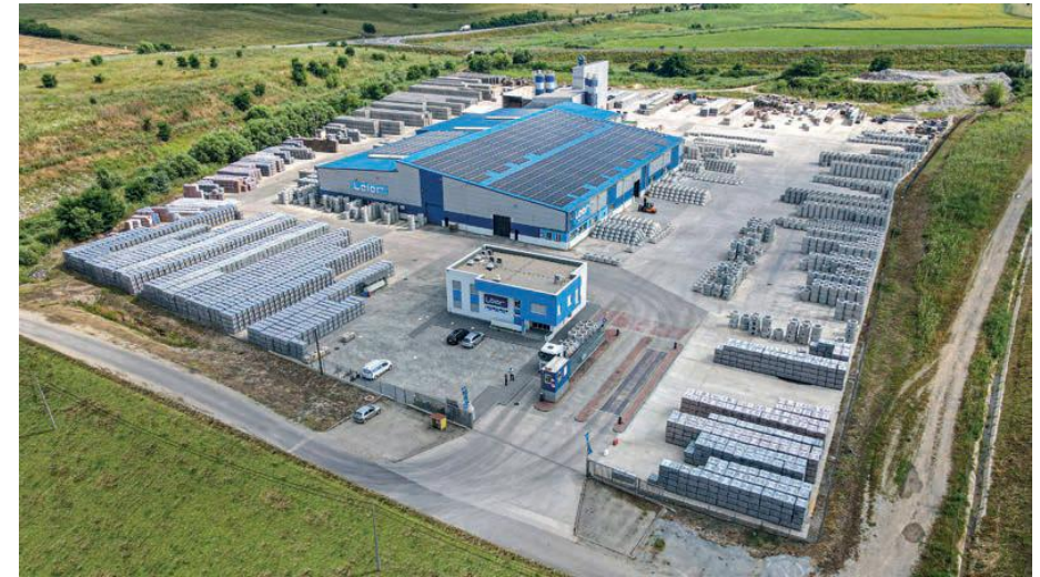
LEIER ROM Unirea (County Alba) plant
