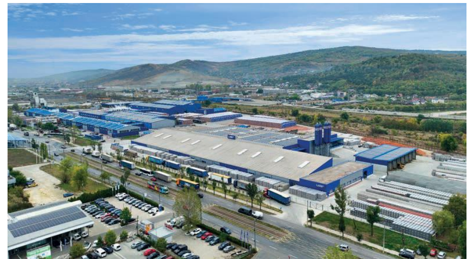
LEIER ROM Iasi Plant
