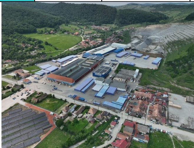
LEIER ROM Sighisoara plant
